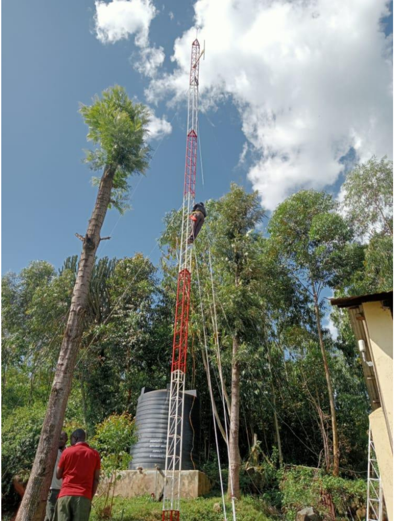
Onyalo radio mast construction in progress
