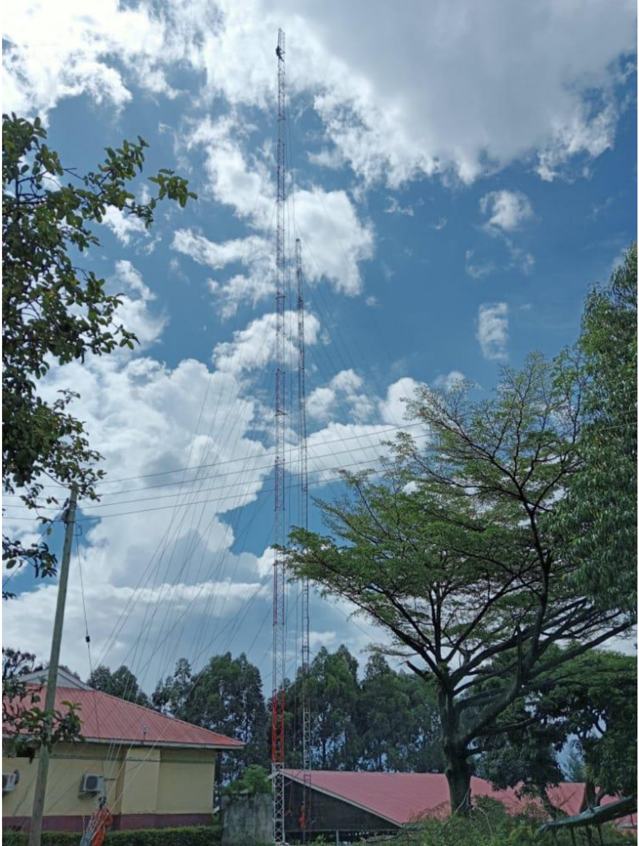
Radio mast at RC HQS in Progress
